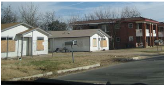
Older Dilapidated Housing Stock
