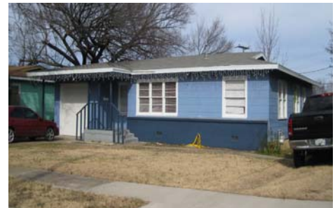
Standard Housing Condition
