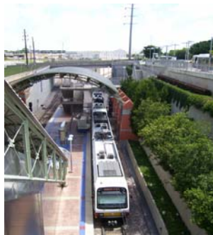
Mockingbird Station, Dallas, Texas
