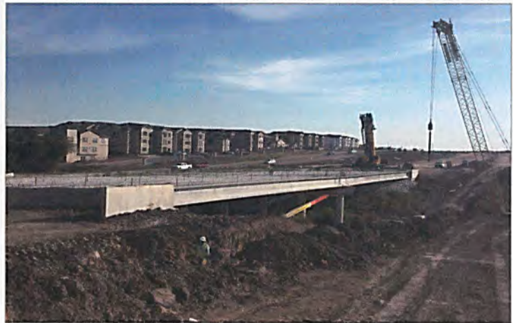
November 2016 - Future SH 360 bridge over Bowman Branch
