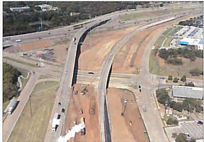
SH 121/360 interchange construction
