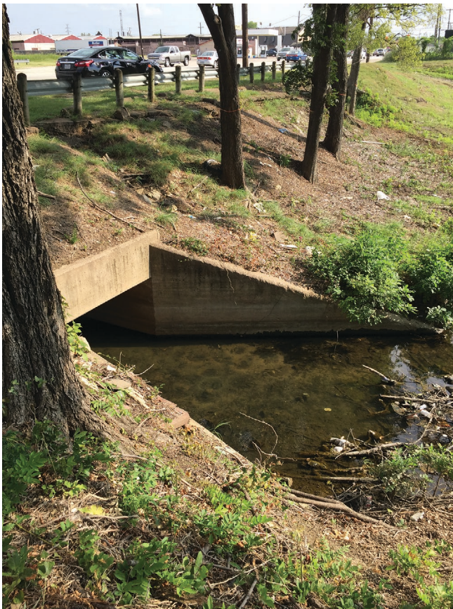
Pond 7 connection to Pond 8
