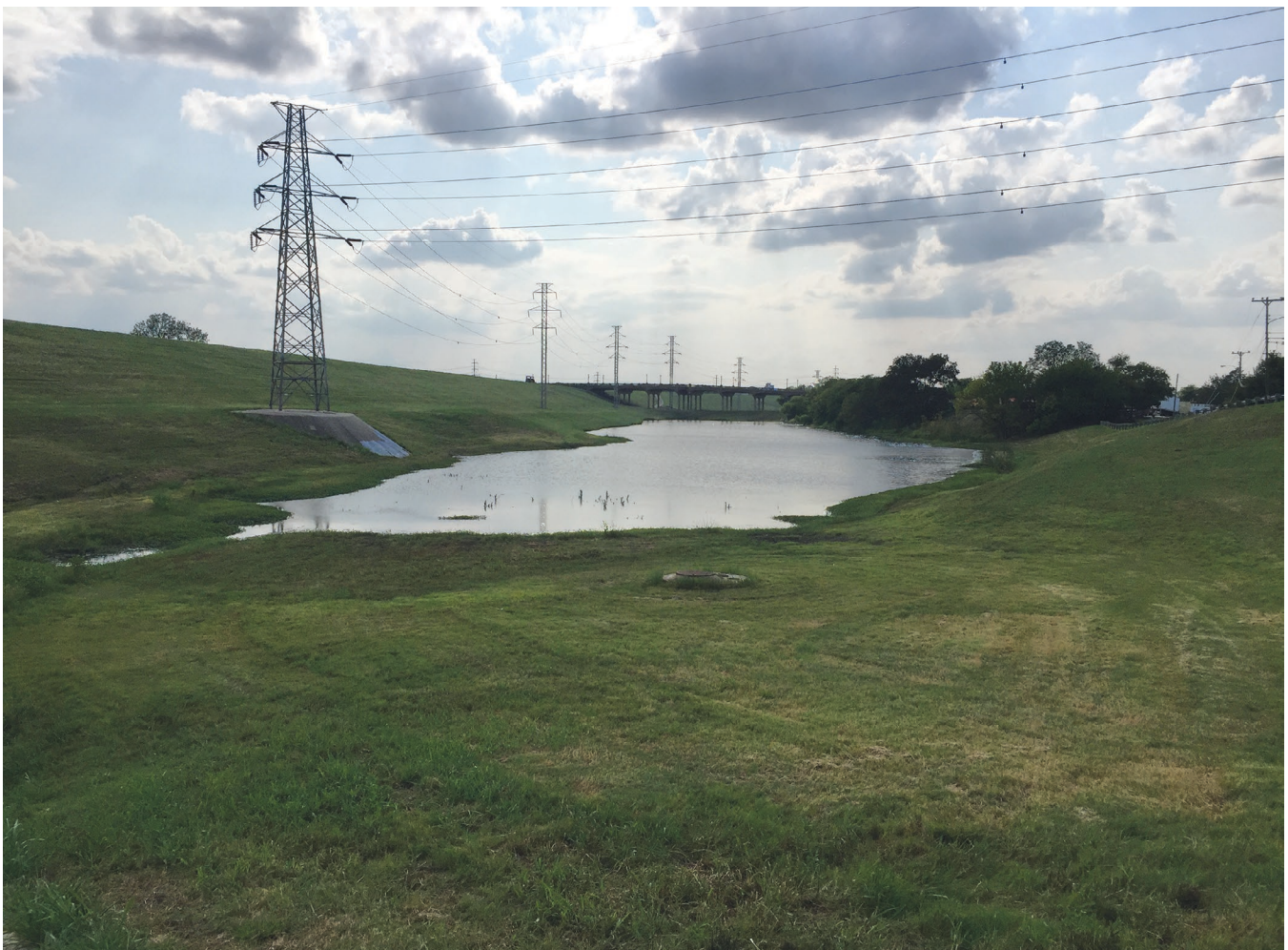
Pond 9 looking west toward the river levee
