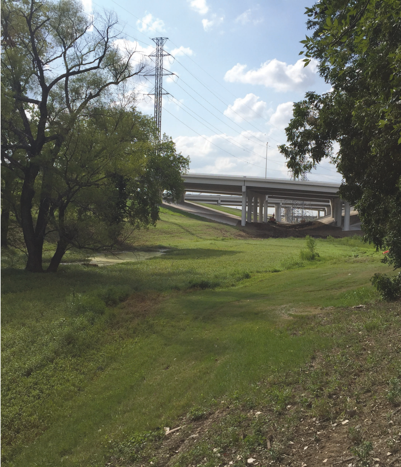
Pond 5 looking northwest toward IH-35 bridges
