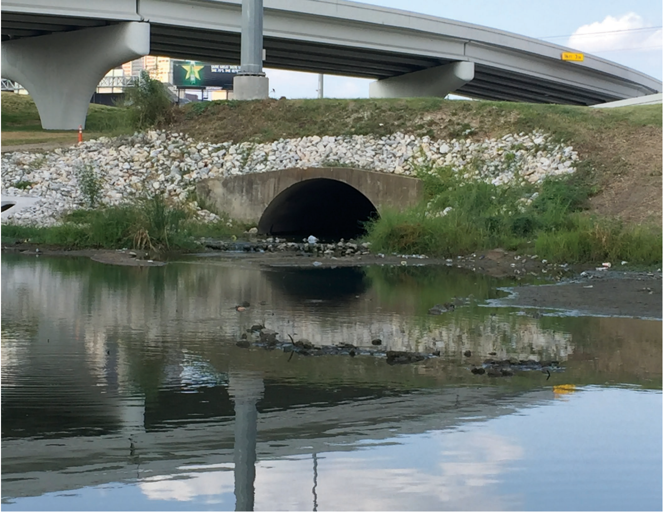
Pond 3 main stormwater outfall
