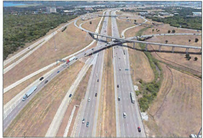
SH 121 at I-635 north of the DFW Airport
