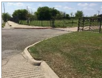
No Sidewalks into Campus
