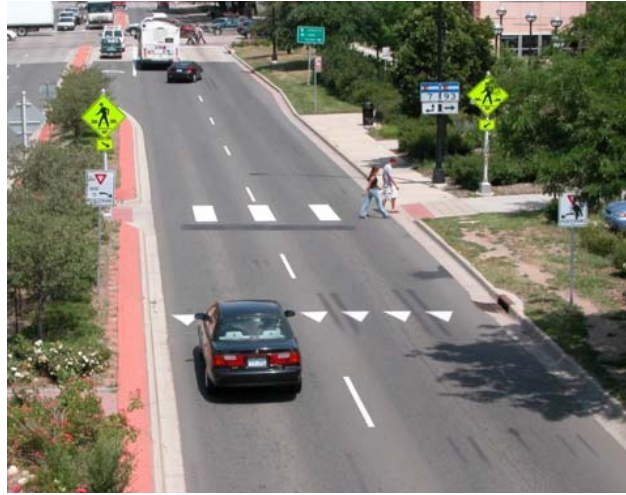
Advance Yield Line and Sign
