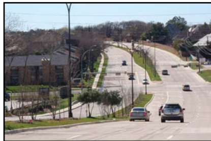
Principal Arterial, 6 Lanes Divided
