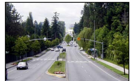
Principal Arterial, 4 Lanes Divided
