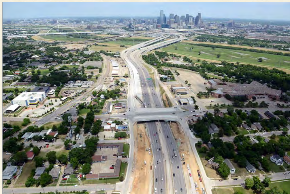
Photo 1: Northbound I-35E/8th Street.
