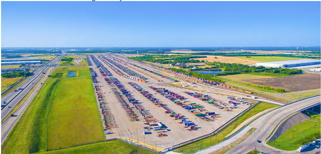
Union Pacific intermodal terminal in Wilmer [Photo: Michael Samples]
