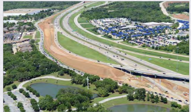
April 2015 -- SH121/360 ramp progress
