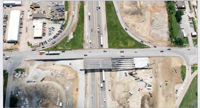
April 2015 -- Expansion work on I-35W at 28th Street.
