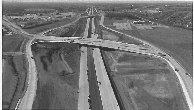
March 2018 - Holland Road and Broad Street bridges over future SH 360
