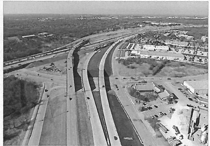
SH 121/360 interchange construction
