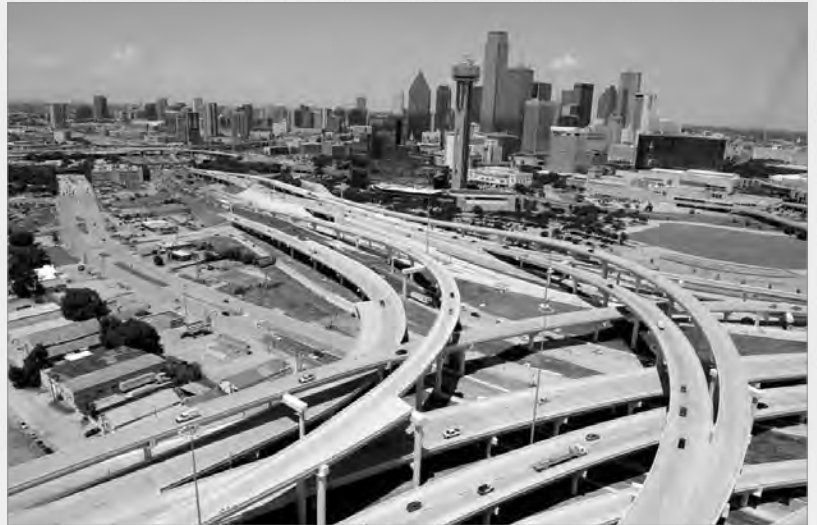
Pictured above: An aerial view of the Horseshoe Project looking east toward downtown Dallas of the new I-30/I-35E interchange.
