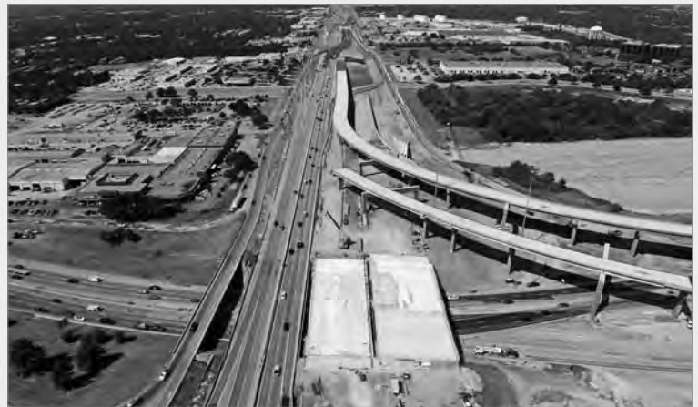
September 2017: Looking west on SH 183 at the Loop 12 direct connections TxDOT photo archive
