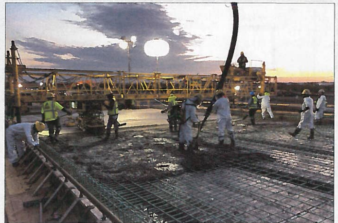
Future westbound I-635 to southbound SH 121 direct connector
