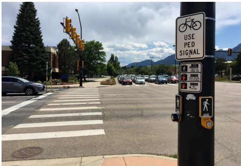
Figure 7. Bicycles Use Ped Signal Sign (R9-5) Installed with Pushbutton
