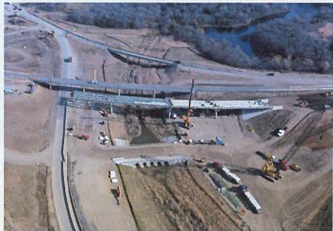
Future I-635 westbound exit ramp to SH 121/FM 2499 northbound
