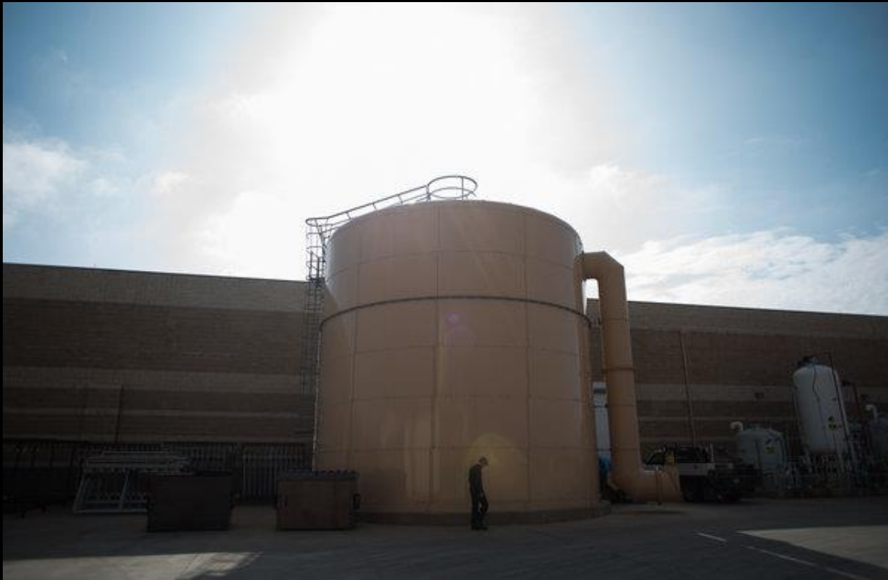
Cypress Water Treatment Plant Wichita Falls
