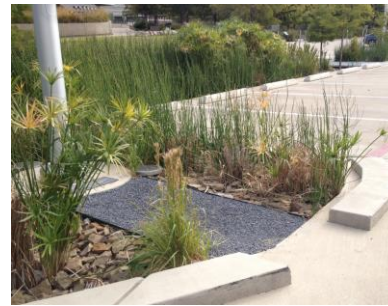
Figure 71. The Perot Museum parking lot bioswales uses native and drought-tolerant plants.
