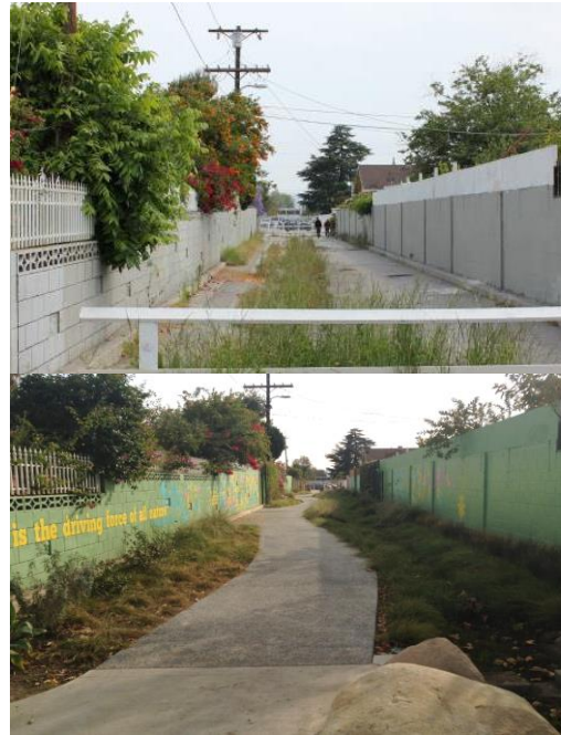
Figure 28. The Elmer Paseo Stormwater Improvement Project transformed an asphalt alley (top) into a green alley (bottom). Source: Council for Watershed Health.
