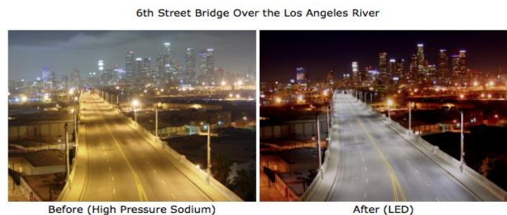
Figure 3. Sixth Street Bridge in Los Angeles before (left) and after (right) the LED streetlight installation.
