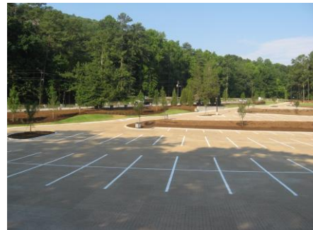
Figure 20. Permeable concrete unit pavers at Triangle Parking Lot in Stone Mountain, Ga. Source: Robert and Company.
