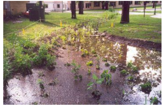
Figure 54. A newly planted bioretention area after a storm.
