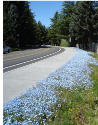
Figure 21. Pervious concrete sidewalk in Olympia, Wash. Source: City of Olympia.
