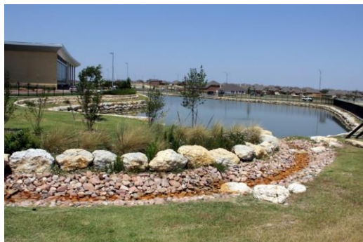
Figure 60. Stormwater pond at Timber Creek High School, Fort Worth, Texas. Source: Teague Nall & Perkins.
