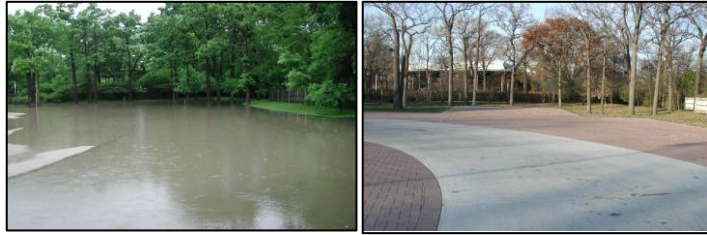
Figure 22. Before (left image, source: Ravinia Festival) and after (right image, source: SmithGroupJJR) the installation of permeable pavers and an underground detention vault at the Ravinia Festival South Parking Lot.
