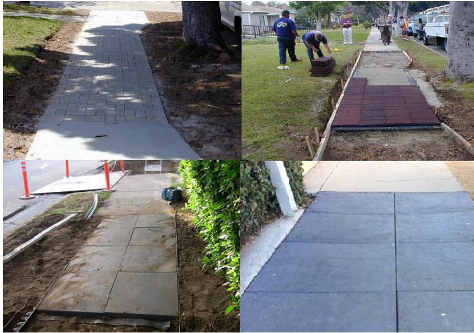
Figure 13. Santa Monica. Top left: brick pavers. Top right: rubber pavers. Bottom left: second-generation TerreWalks. Bottom right: third-generation TerreWalks. Source: City of Santa Monica, Calif.
