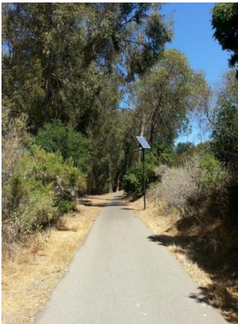
Figure 6. Solar lighting used in the Obern Trail Retrofit Project, Santa Barbara, Calif. Source: County of Santa Barbara.
