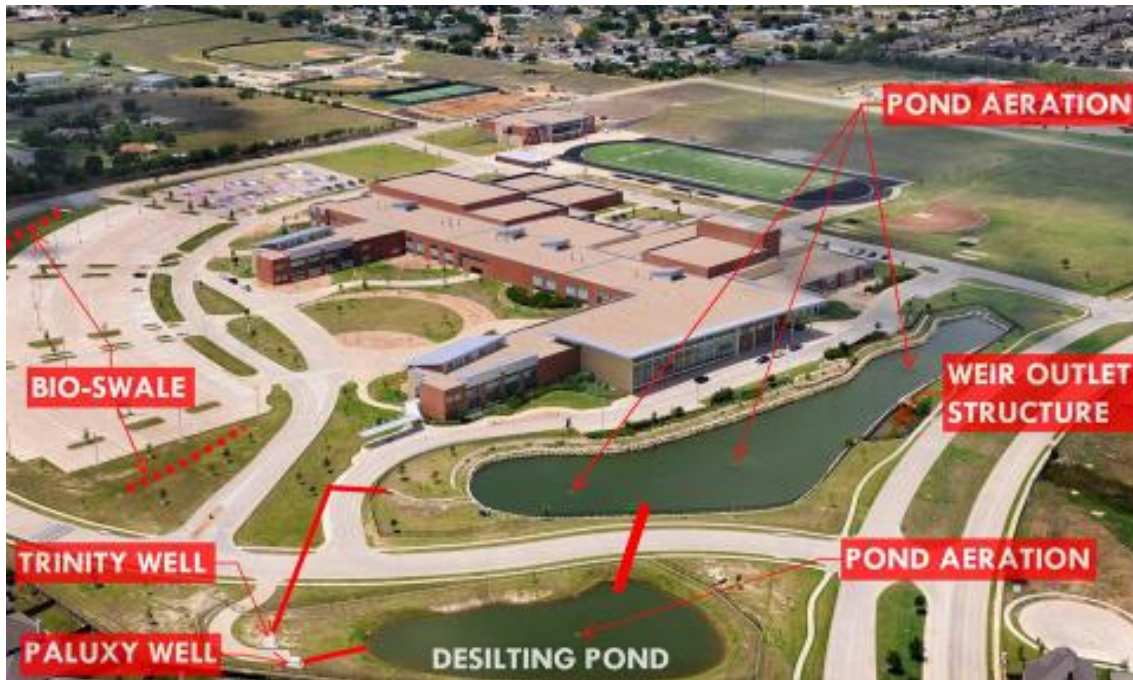
Figure 34. Green infrastructure elements at Timber Creek High School, Fort Worth, Texas. Source: Teague Nall & Perkins.
