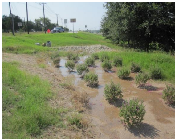
Figure 63. Bioretention pilot in Bryan, Texas. Source: Texas A&M University/Texas A&M Transportation Institute.
