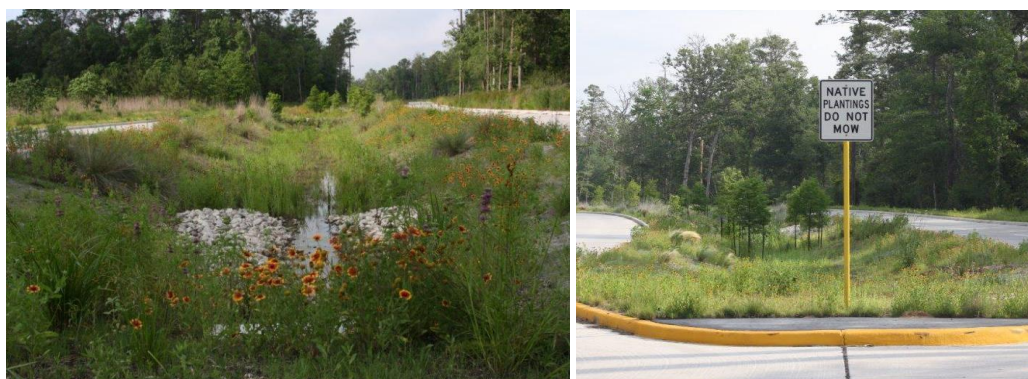
Figure 66. Green stormwater infrastructure at Birnamwood Road.
