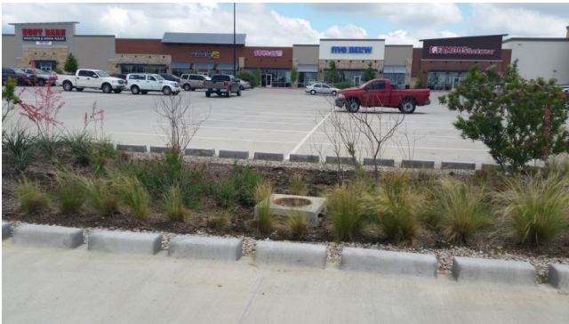
Figure 31. Parking lot island with sawtooth curbs at Rayzor Ranch North, Denton, Texas. Source: Dunaway Associates.
