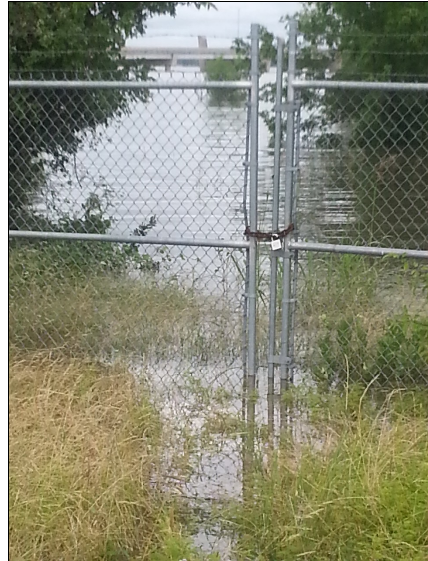
Plant Outfall channel Looking toward Toll Bridge
