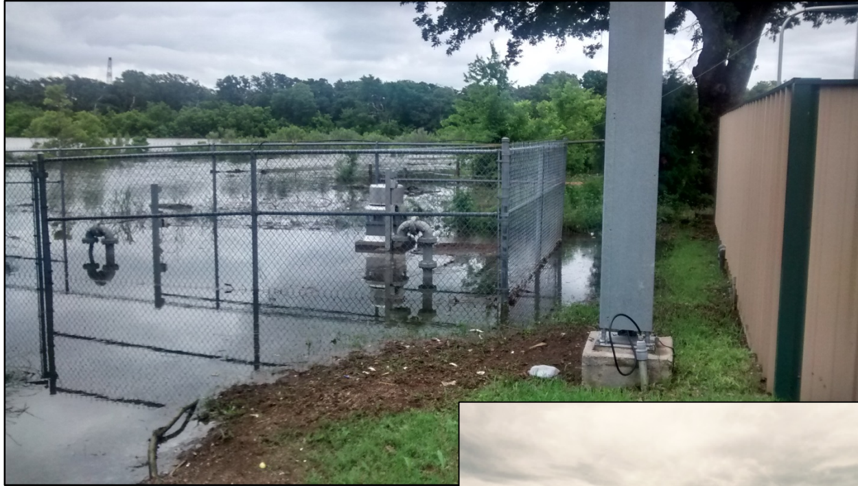
Meter vault submerged
