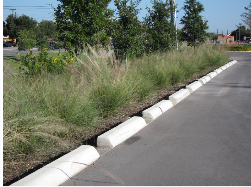
Bioretention Facility in San Antonio, TX. Source: Tetra Tech
