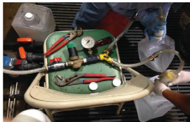
Plant Operators Collecting Compliance Samples
