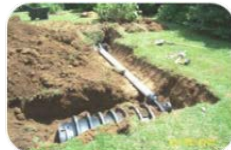
Stormwater and Infrastructure
