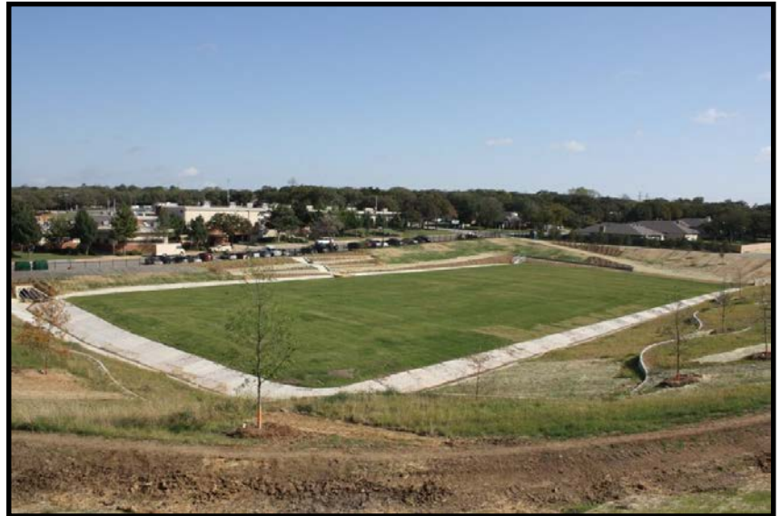
Multi-Use Detention Basin & Athletic Field at Eastern Hills Elementary School- Partnership with Fort Worth ISD
