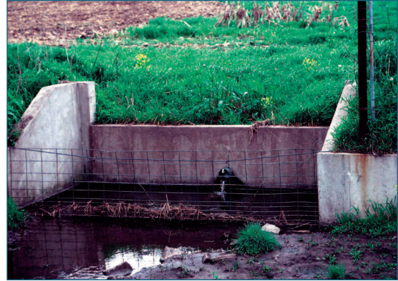
Figure 6. Grade stabilization structure. (Source: USDA–NRCS)
