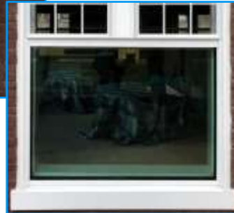
Before Faux Mullions
