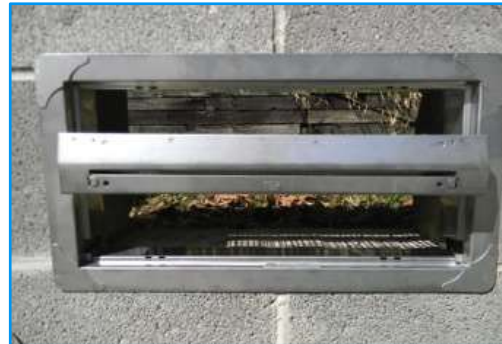
Flood door activated, reveals an unobstructed opening.
