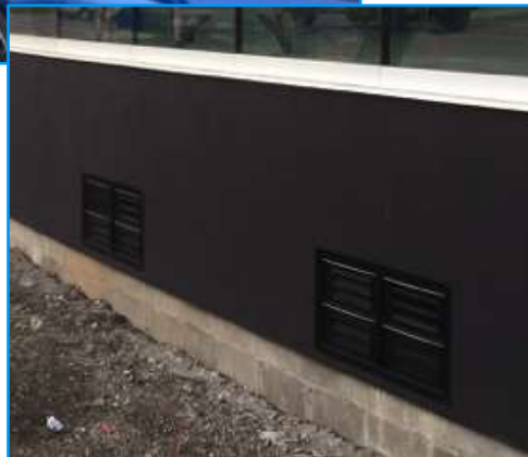
2x2 Multi-Frame 800 sq. ft. of flood protection each
