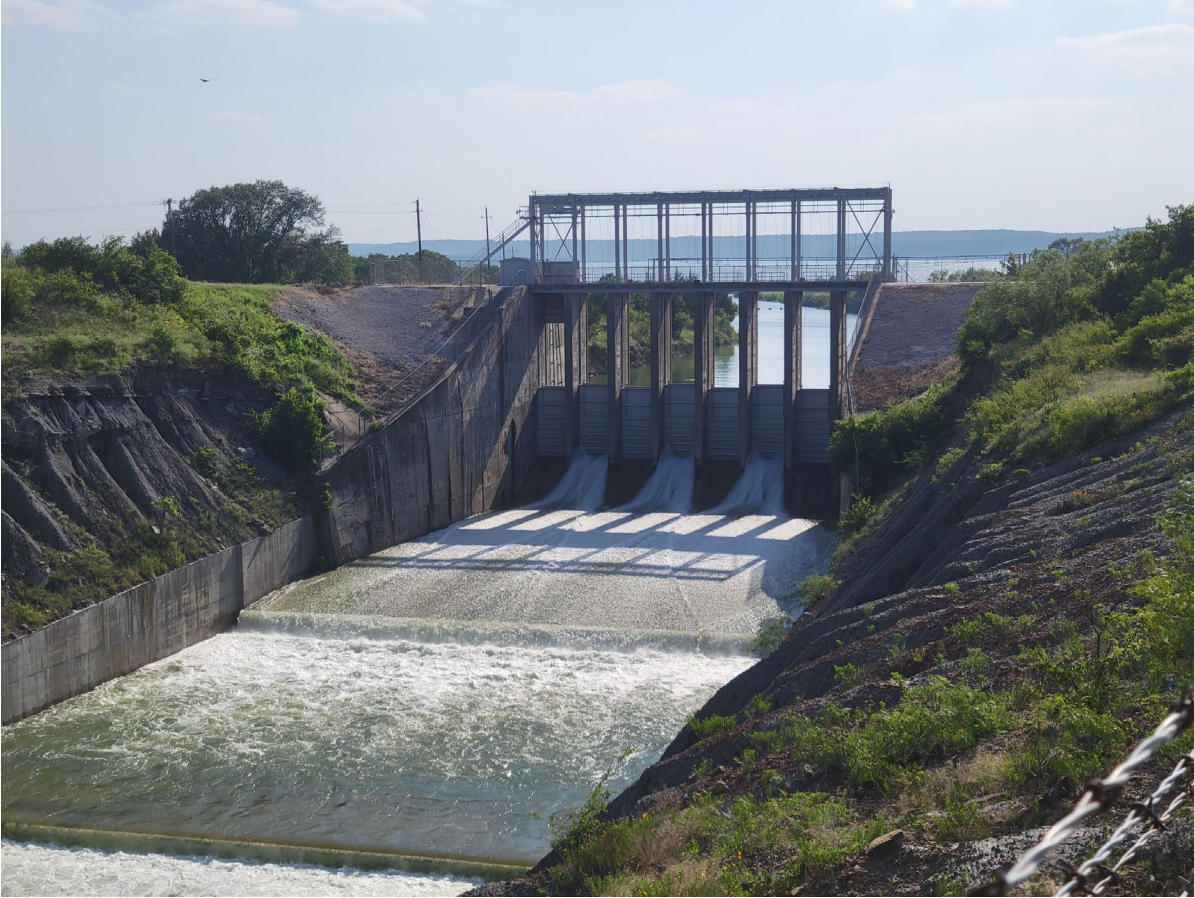
2021 Lake Bridgeport Spillway (Source: TRWD)
