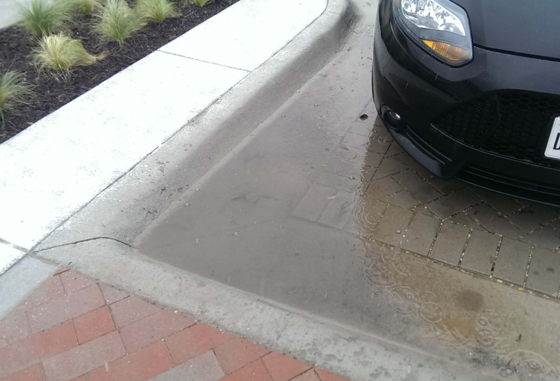
Hickory Street – Interlocking Pavers
