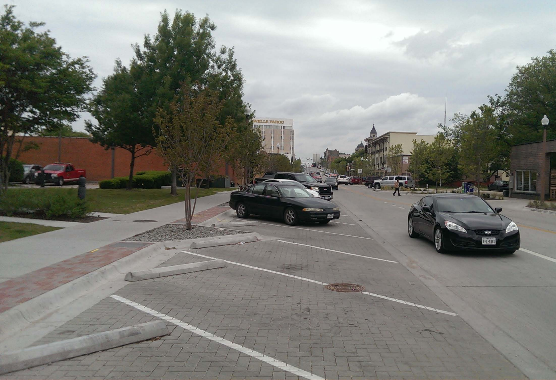
Hickory Street – Interlocking Pavers
