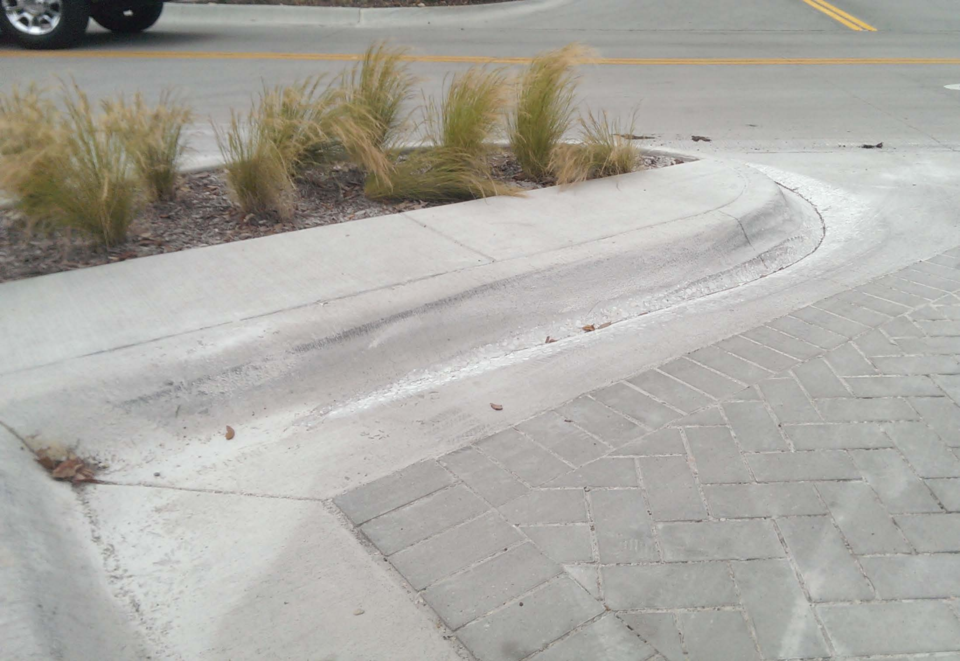
Hickory Street – Interlocking Pavers
