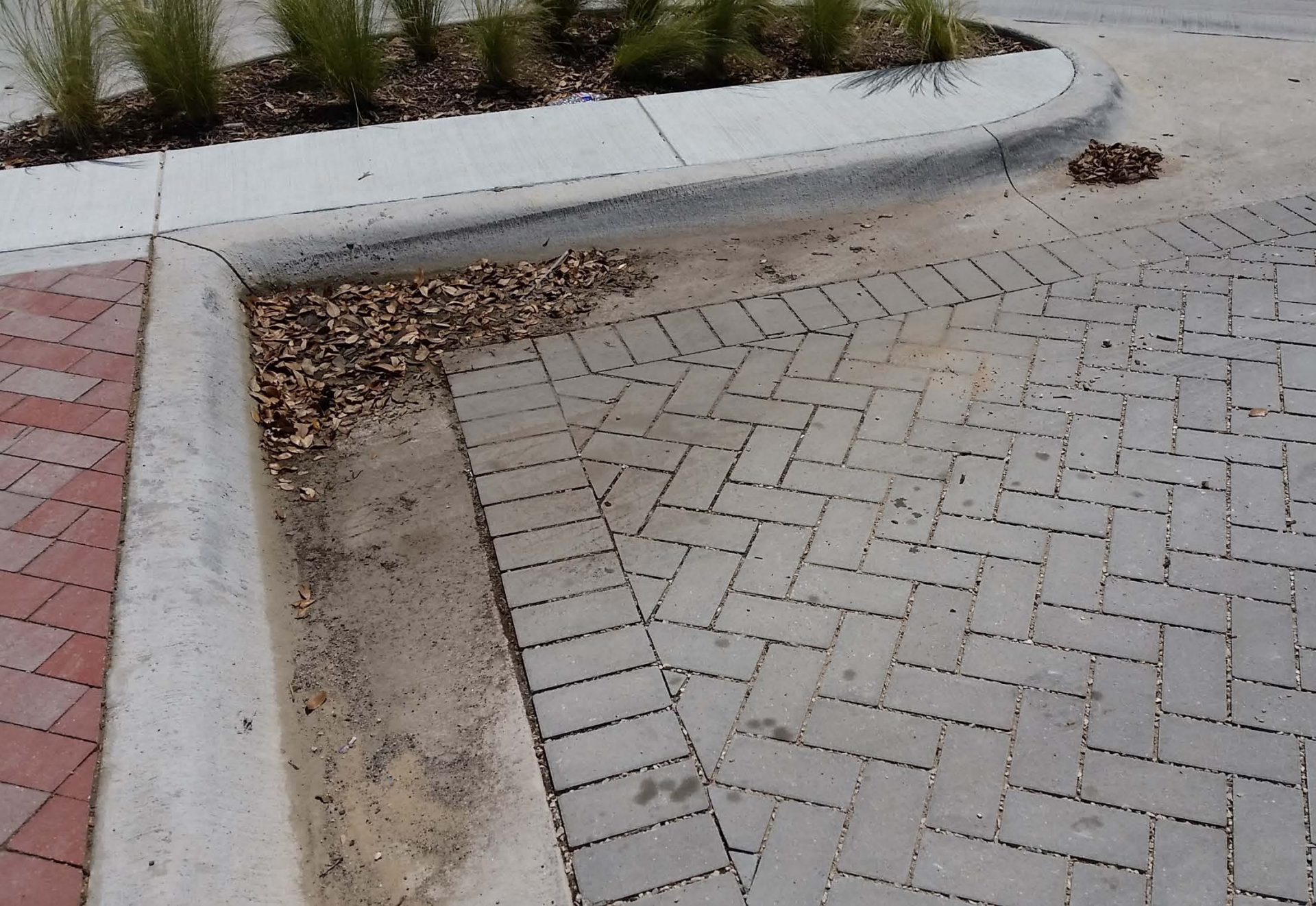
Hickory Street – Interlocking Pavers
